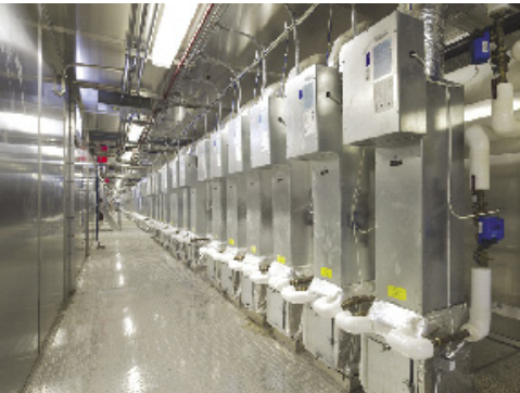
Roof top maintenance tunnel
